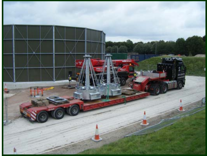
Delivery of HYCOVER Centre Columns.
