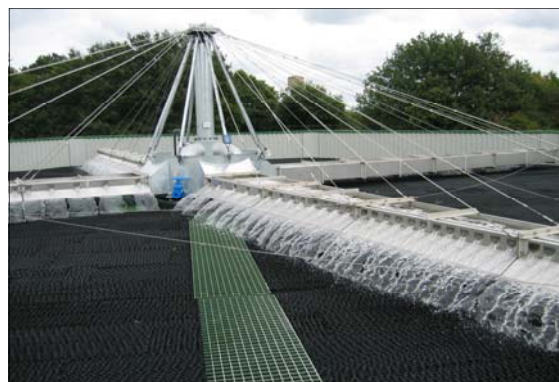
4 Arm motor driven HYCOVER trough arm distributor applying some 360 lt/sec to 20.0 mt dia HYRATE nitrifying filter.
