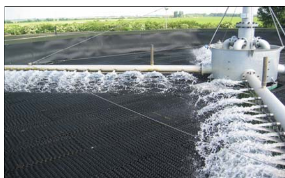
4 Arm motor driven HYCOVER tubular arm distributor applying some 170 lt/sec to 12.0 mt dia HYRATE nitrifying filter.
