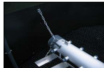
Distributor arms are fitted with Quick strip full flow washout end cap & stainless steel chain..
