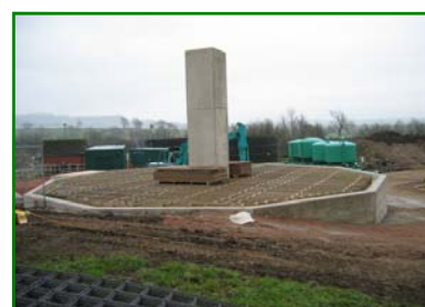
Timber matrix modules in place ready for construction of new HYRATE Polytower filter shell.
